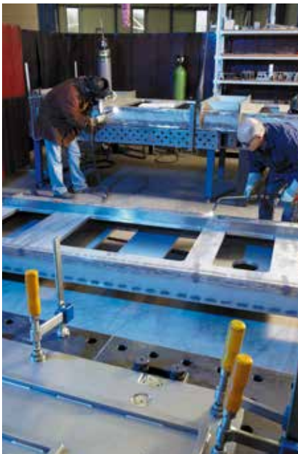
Warping due to welding and machining is corrected with precision on our jigs and fixtures.
