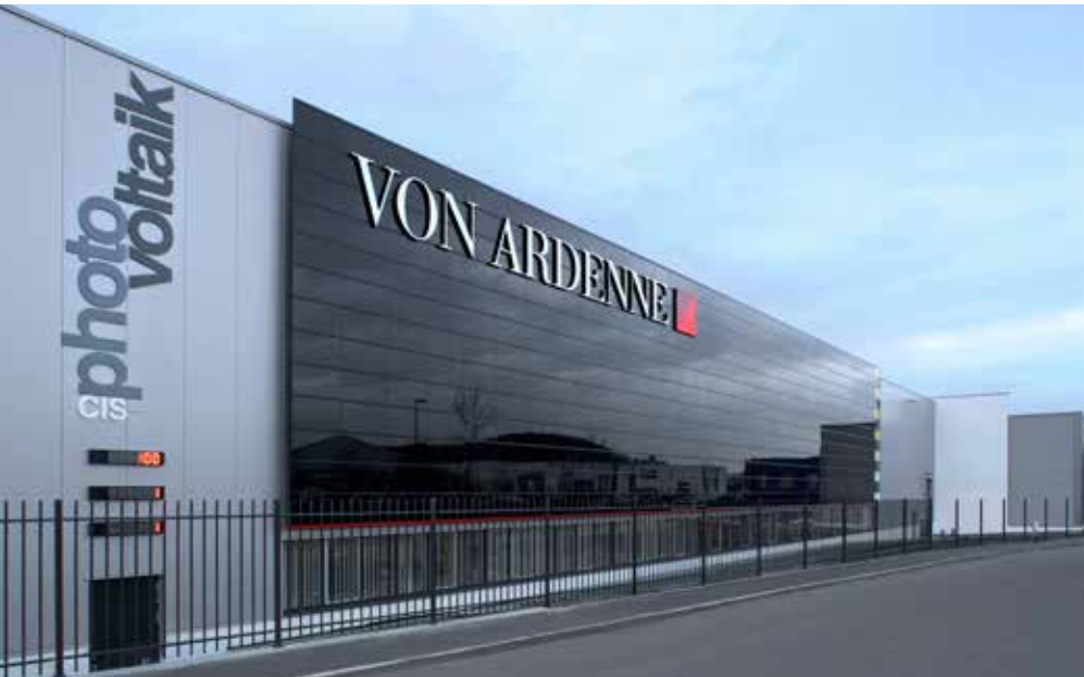
VON ARDENNE GmbH production shop with thin-film photovoltaic modules on the façade. (Photo: VON ARDENNE Corporate Archive)
